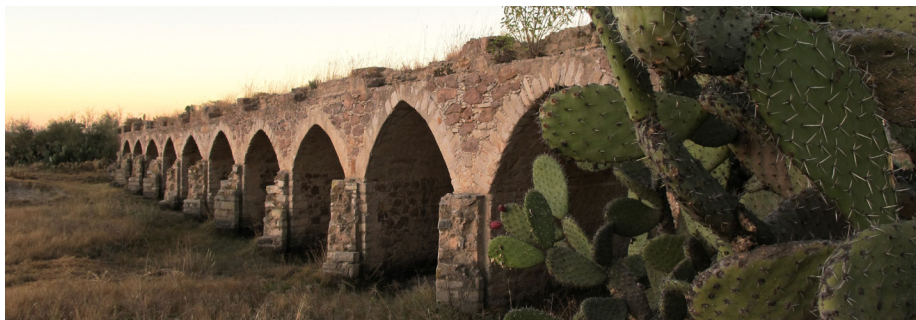
Bridge of Ojuelos, State of Jalisco, Mexico
