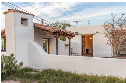
Restored Casa Ortiz, Socorro
