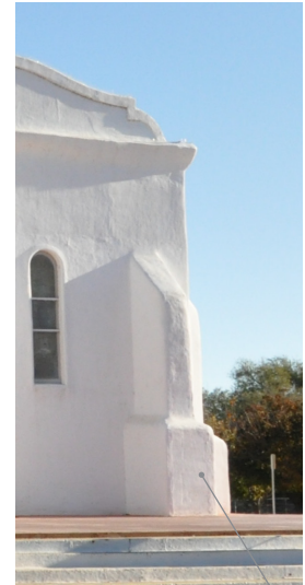
buttresses and wing walls
