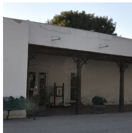
Typical roof in the San Elizario Historic District with scuppers, parapet roofing and wooden porch
